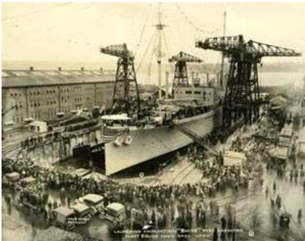
An Ammo ship being built , Puget Sound, 12/16/1919
